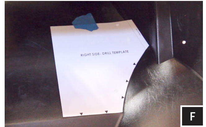
F. Cut out the RIGHT template along the cut line. Position the template on kick panel in the passenger footwell above the foot rest making sure to line up arrows on template to the curves of the panel as seen on image F.
